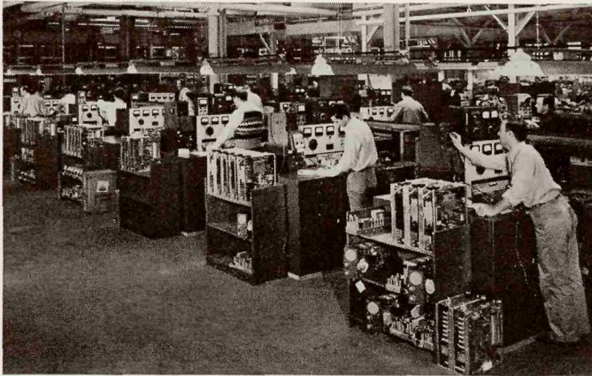
Phasing communications equipment
