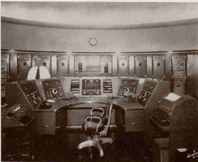
Control room for two-way radio communications system.
