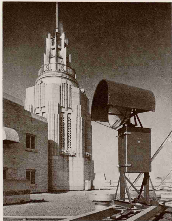
Microwave transmitting unit atop a tall building.
