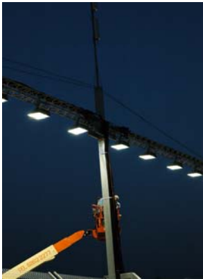
Antenna installation on a light tower
